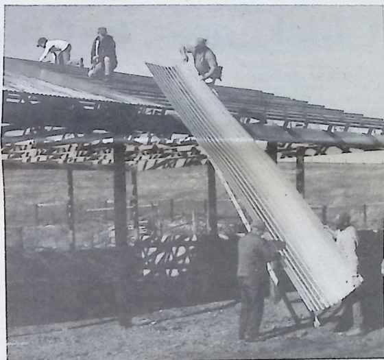
Step 4 — The metal sheeting goes on the roof.
