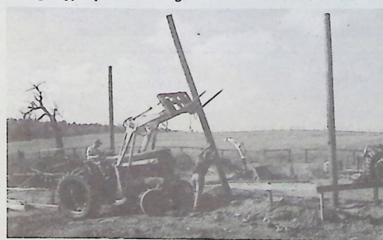
Step 2 — Posts, those left behind on our property by the utility company when power lines were upgraded, were set, creating our own version of Stonehenge, above right.
