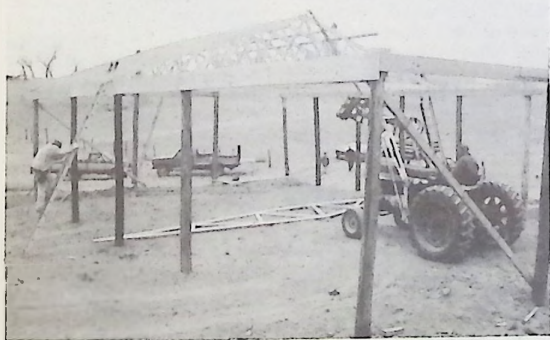
Step 3 — The top band and roof trusses are set. A neighbor loaned us a special tool that fits over the bale spear on the tractor's front-end loader to help place the trusses.
