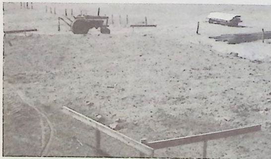
STEP 1 — Forty-four tons of ground up road surface that a paving company was trying to get rid of was used for fill to make the pad for the machine shed. A 56x36 area was measured off designating the base of the shed.
